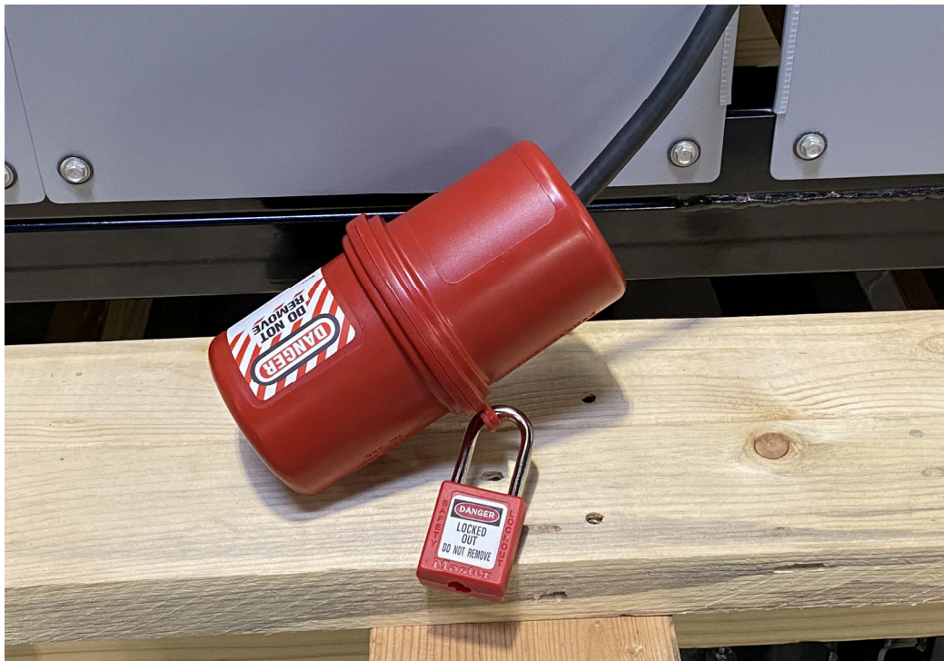
Figure 2: Lockout of Electric Motor Machines
